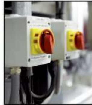
Motor disconnect
